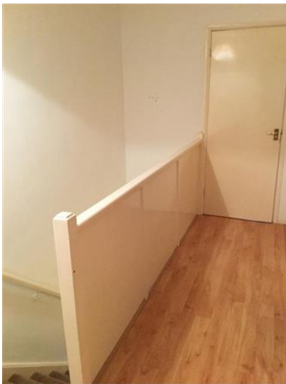
Stair and landing clean and tidy
