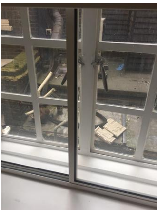
White painted critall windows, single glazed, silver frame Secondary glazing
